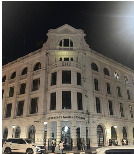
Figure 2. London Sumatra Building (Lonsum)
