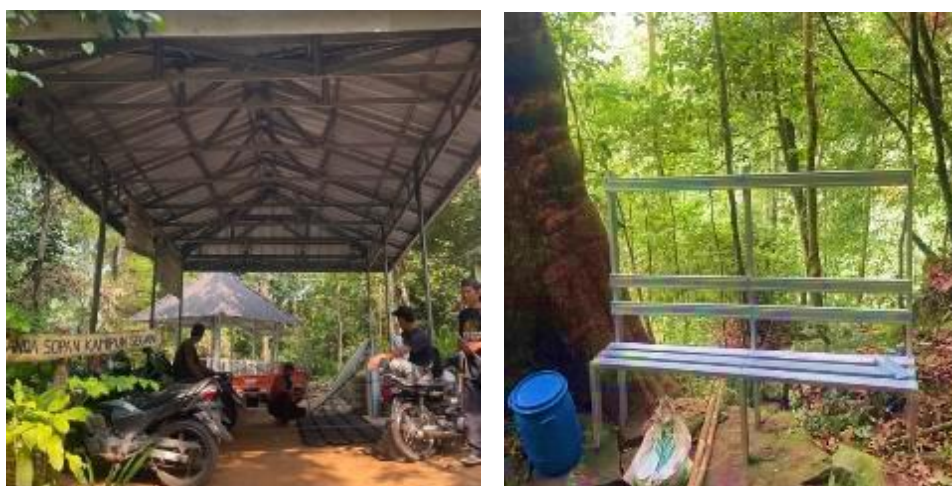
FIGURE 3 & 4. Construction Process of Facilities on the Indukan Waterfall Route Source: Astriyantika, dkk (2024)
